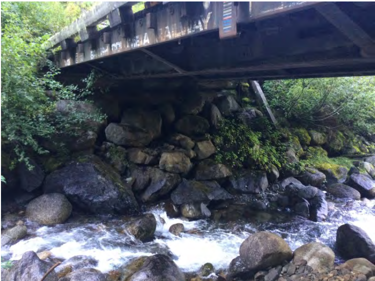
Left Bank Abutment when facing downstream
