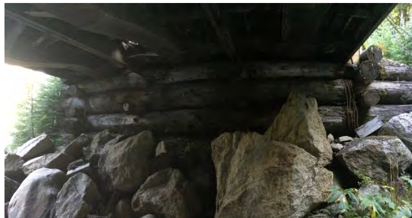
Right Bank Abutment when facing downstream
